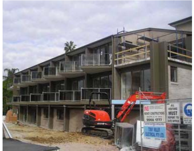
Ashburn House with distinctive triangular decks, under construction
