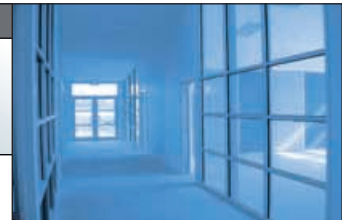
USG Powerscape 13mm linings are used throughout this school classroom block.
